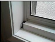
Reveal DAMAGE, impact damage, over paint, Right wall.
