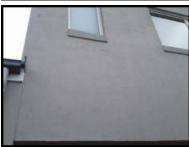
Mortar Cladding marks, dirty, paint starved, south elevation.
