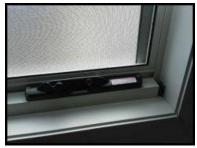
Woodwork Architrave mitre poorly finished, window.
