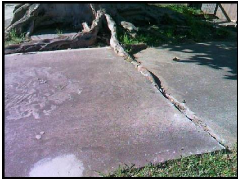
Crack Type: Differential movement cracking Width: 15mm Length: 3.0M.
