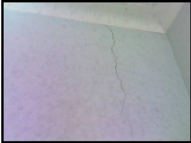
Crack Type: Differential movement cracking Width: 15mm Length: 3.0M.
