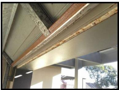
Front Doors - Type & Condition: The main garage door is a panel lift style door and is in fair condition.
